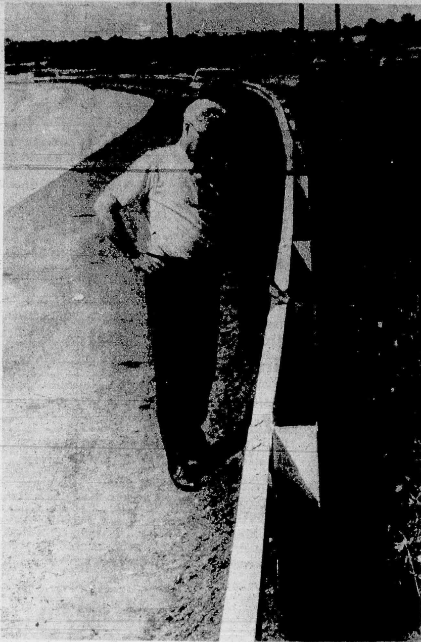
MORE POSTS - Mayor Ken Smith inspects new guardrails placed along Route 21's "Death Strip" in Belleville. Besides raising the rails, the state placed the steel posts you see here at six foot intervals instead of 12 feet intervals. (please see story on page one)
