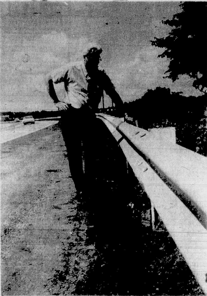
SAFETY IMPROVEMENTS — Mayor Ken Smith inspects higher guardrails installed by State Highway Department on Route 21's "Death Strip." Dirt mounds in front of rails were scraped to road level in an effort to prevent cars from "flipping over the rails and into the Passaic River."
